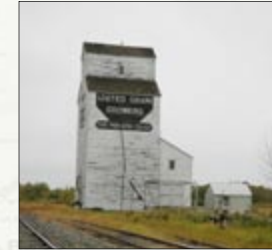
Single elevator, Kinuso
